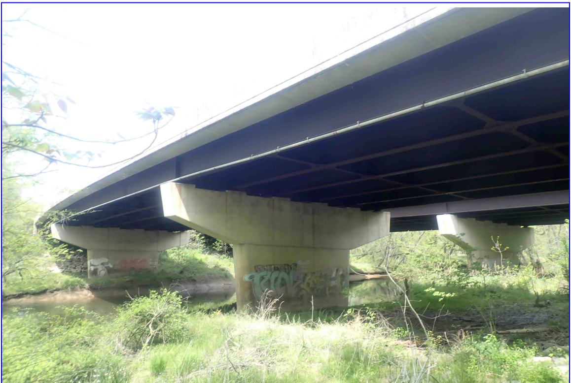
2. SOUTH ELEVATION LOOKING NORTHWEST
