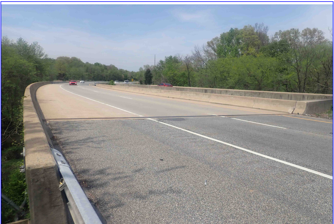
6. CONCRETE DECK & ASPHALT COVERED EAST APPROACH SLAB LOOKING WEST
