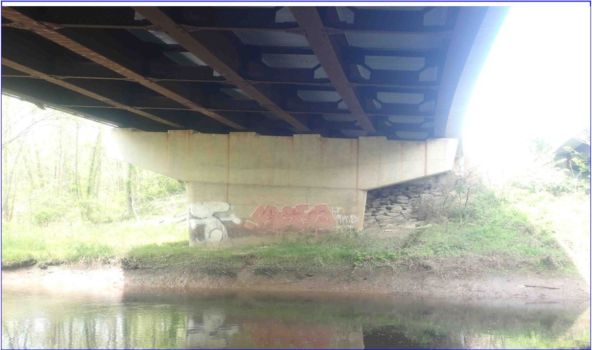
3. GENERAL VIEW OF SPAN 2, PIER 1 LOOKING WEST
