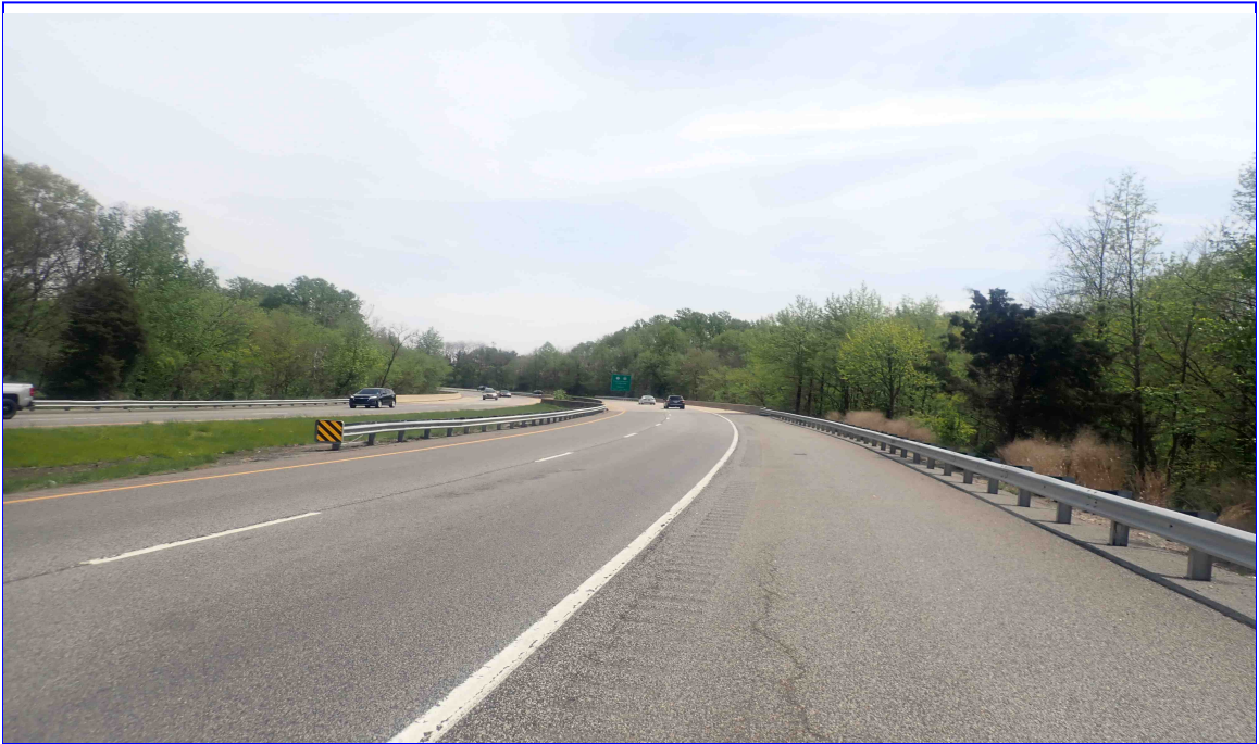
1. WEST APPROACH ROADWAY LOOKING EAST
